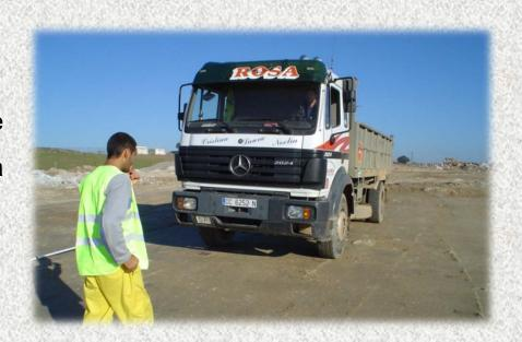
☐ Compaction control procedures revised: wheel impression test, topographic settlement, plate load test.
